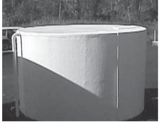
Fiberglass tanks offer solid covers. The fiberglass must be cured on the inside to avoid bad tasting water. The tanks can be made of food-grade materials, so no liner is necessary.
