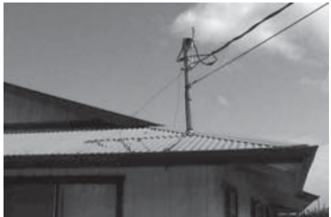
Rodents can access your roof by climbing utility poles and running along electrical and phone cables. Putting the wires underground is an expensive but good solution to the problem. Attaching the wires to the side of the house may be an option if the house is tall enough to keep the wires out of reach. Contact your utility companies for advice.
